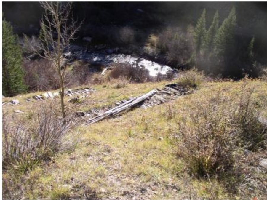
What is left of the Upper Trestle (Bridge 57A) on the uphill side. This shows the remains of two sill beams – that supported two of the 20 trestle bents – resting on stone piers.
